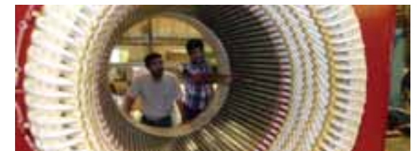
Rewinding of 16000HP Stator for Saudi Aramco
