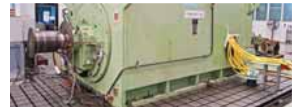
Overhaul & repair excitation system of 25000HP, 13.2KV, 1800RPM motor
